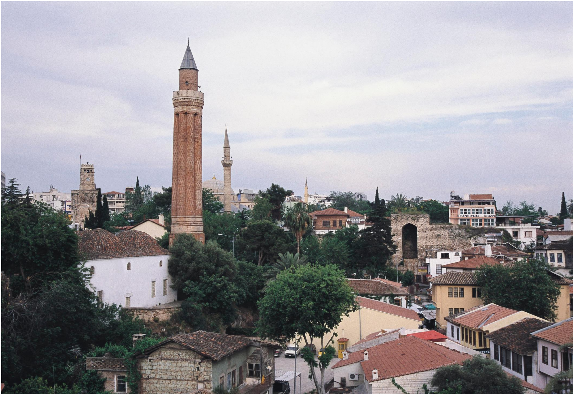
Yivli Minarete- Clock Tower
